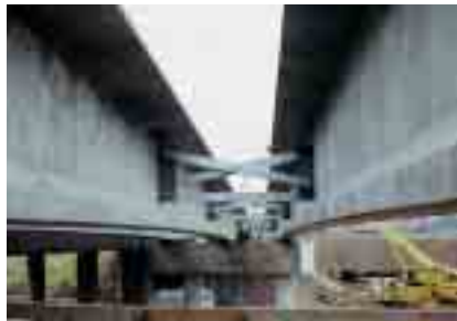
The S.R. 741 overpass over I-71 in Cincinnati, was redesigned to feature continuous bulb-tee beams. The project is one of the first in the state to use precast bulb-tee beams on an interstate overpass.
