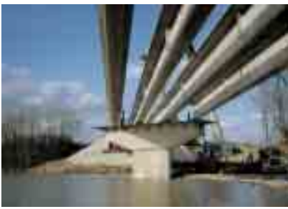
Now being completed, the Souder Avenue Bridge over the Scioto River in Columbus, Ohio, features three spans using continuous bulb-tee beams and hammerhead piers.
