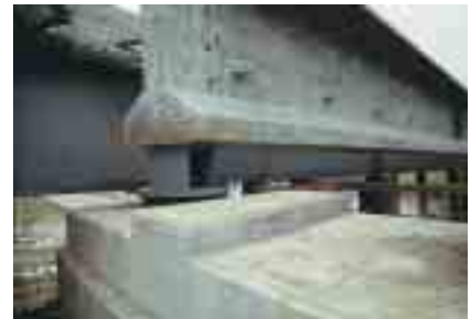
The S.R. 741 overpass over I-71 in Cincinnati, was redesigned to feature continuous bulb-tee beams. The project is one of the first in the state to use precast bulb-tee beams on an interstate overpass.
