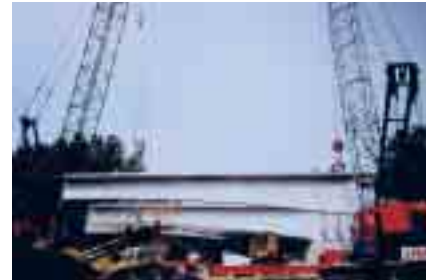
The Third Avenue Bridge design incorporates two 135-foot spans comprising 28 variable-depth post-tensioned spliced bulb-tee beams, each 67'4" long.
