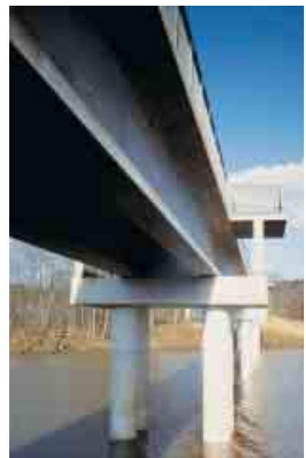
The pedestrian bridge over Winton Woods Harbor in Cincinnati, was redesigned to use 90-foot precast bulb-tee beams, which reduced the number of original beams by 33 percent.
