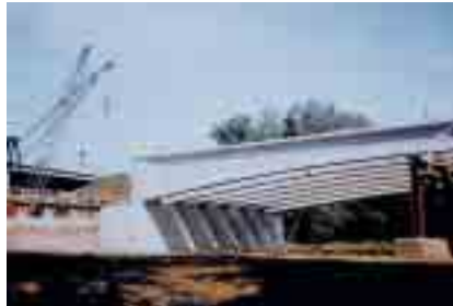
The Third Avenue Bridge design incorporates two 135-foot spans comprising 28 variable-depth post-tensioned spliced bulb-tee beams, each 67'4" long.
