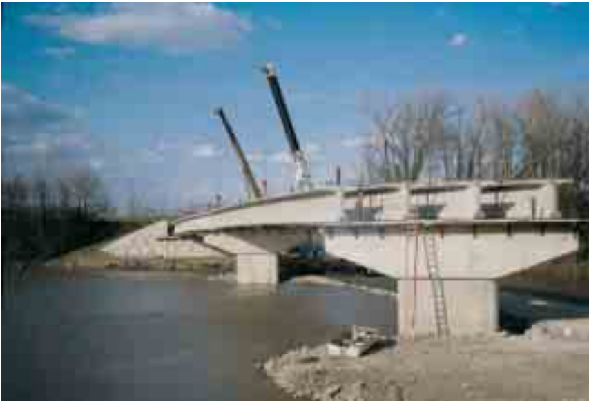
Now being completed, the Souder Avenue Bridge over the Scioto River in Columbus, Ohio, features three spans using continuous bulb-tee beams and hammerhead piers.
