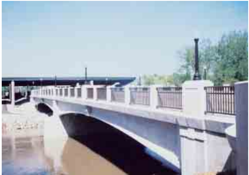
The Third Avenue Bridge over the Olentangy River located in Franklin County, Columbus, Ohio, features a variable-depth post-tensioned spliced bulb-tee beam, the first of its kind to be used in the state.
