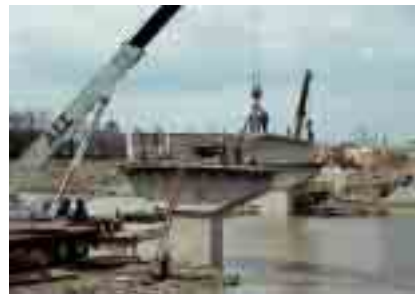
Now being completed, the Souder Avenue Bridge over the Scioto River in Columbus, Ohio, features three spans using continuous bulb-tee beams and hammerhead piers.
