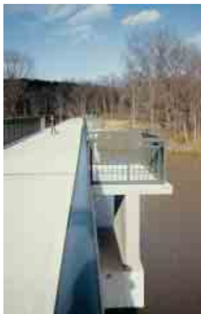
The pedestrian bridge over Winton Woods Harbor in Cincinnati, was redesigned to use 90-foot precast bulb-tee beams, which reduced the number of original beams by 33 percent.
